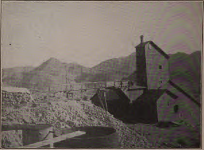
Mill for Concentrating Lead Ore, Quitman Mts., El Paso County
